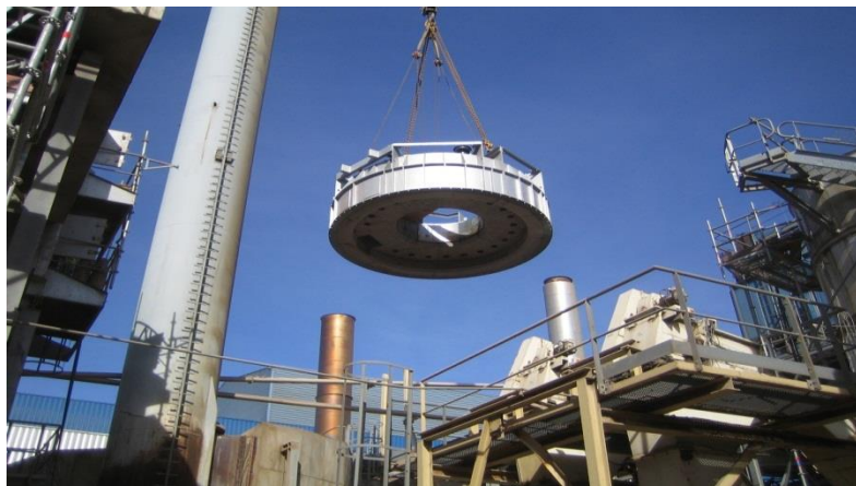
New roof for existing combustion chamber
